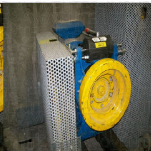
La machine de traction.
